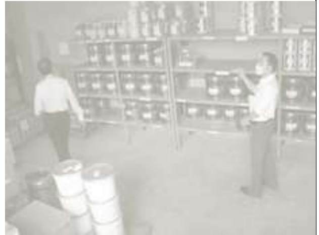
Dangerous goods storage area
